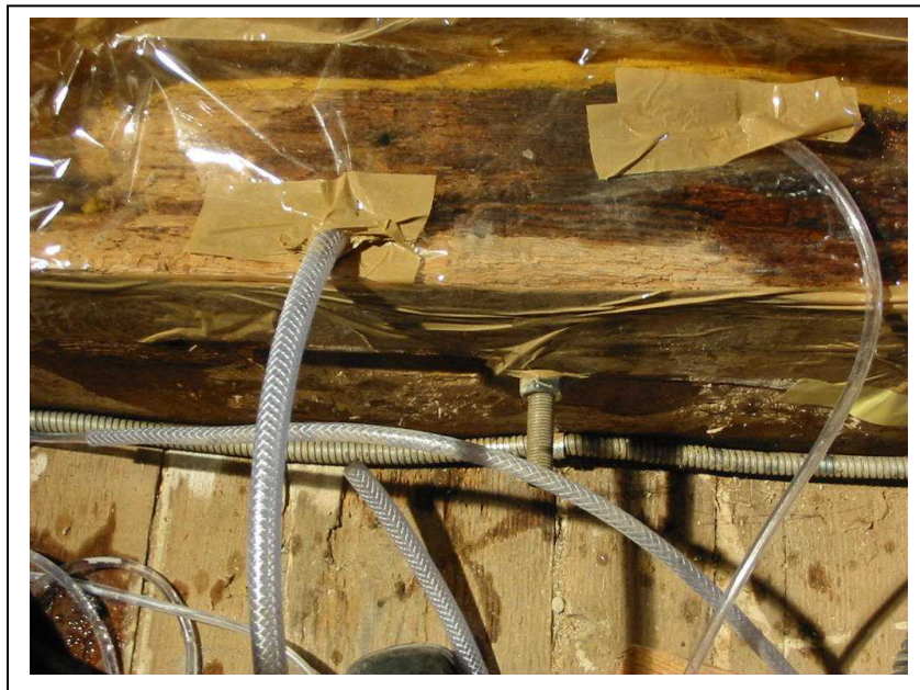
Figure 2. Vacuum consolidation of wooden prop (girders).
