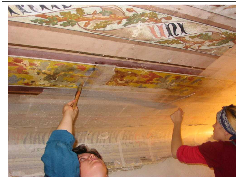
Figure 4. Consolidation of coloured layers.
