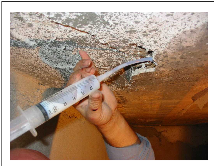
Figure 5. Consolidation of prop detachment (intonaco).
