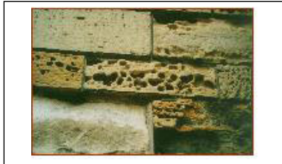
Figure 5. Details with stone and cement plating from the 1906-1908 restoration (the south facade). Humidity effects.
