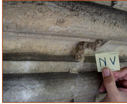
Figure 3. Deposits of dust – mud and vegetal material and film of soiling.
