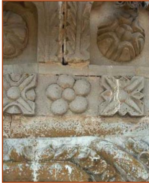
Figure 2. Soiling by droppings from birds and biological colonization.
