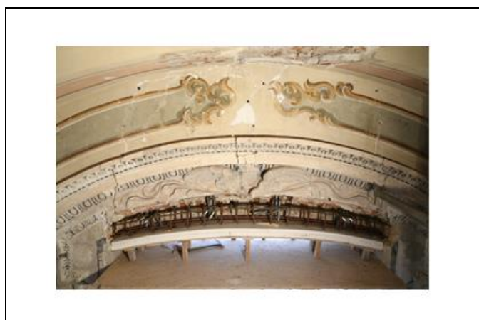
Figure 6. Reinforcement of the window lintel by using steel construction.
