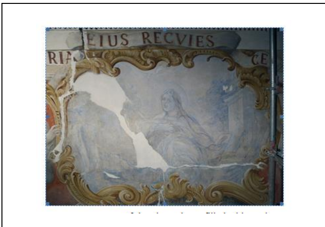
Figure 12. Loses of the plaster layer filled with putties.
