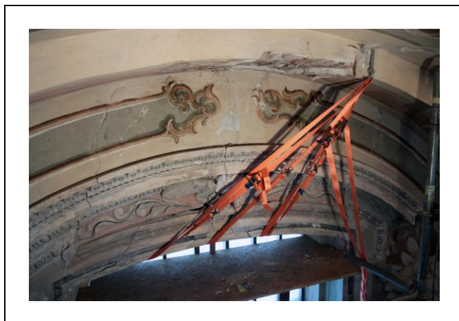
Figure 5. Temporary protection of the window lintel by using belts.
