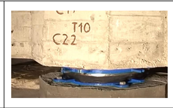
Figure 9. Seismic isolators
