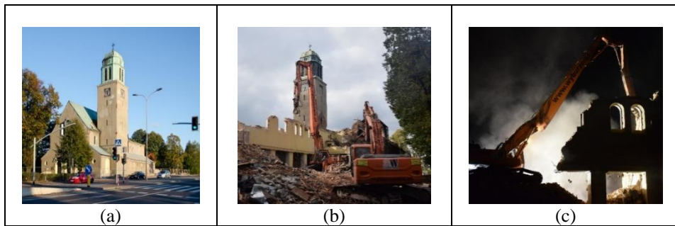
Figure 6. Church of St. Joseph the Worker in Bytom – designed by Theodor Ehl, 1928-2016 (a), Demolition of the Church of St. Joseph the Worker in Bytom – 2016 (b, c).
