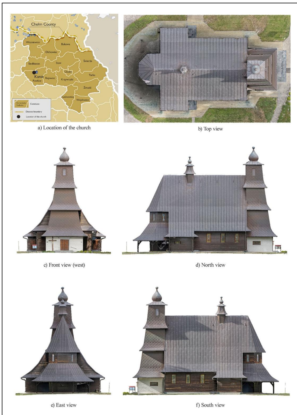
Figure.11. Architectural inventory of the church in Kania - photogrammetric method: a - Location of the church; b – f - Inventory materials of the church in Kania (2024); source: a – map by K. Kluz; b-f - photogrammetry by M. Wac
